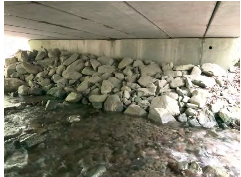
Left Bank Abutment when facing downstream
