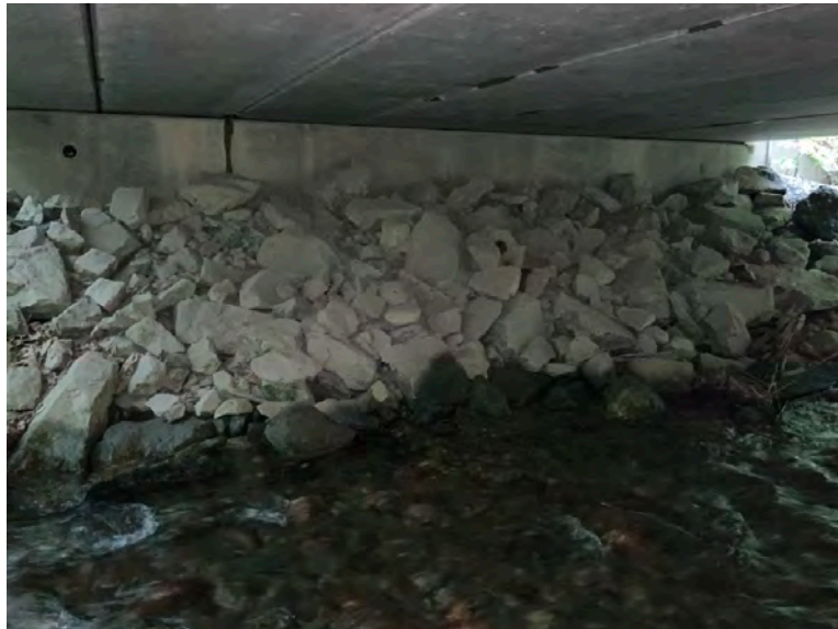
Right Bank Abutment when facing downstream
